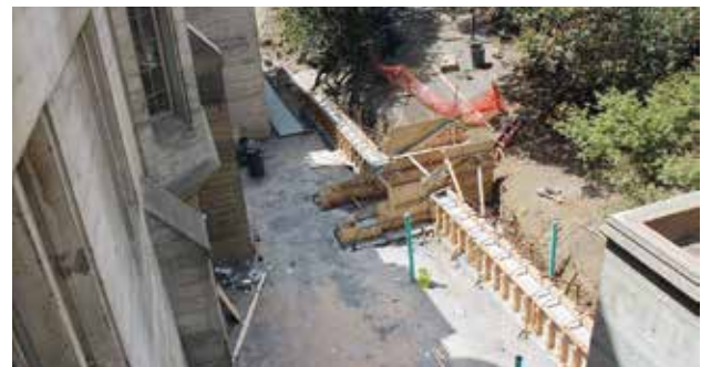
Requiring substantial seismic retrofitting, the back patio will now literally support the rest of the Hall in event of an earthquake.
